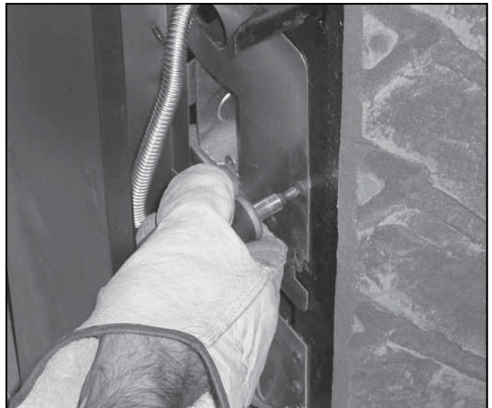
Figure 13.3 Remove Access Panel Screw
